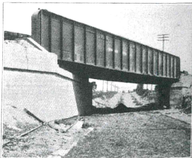
Highway Under-Crossing on a Sharp Skew
